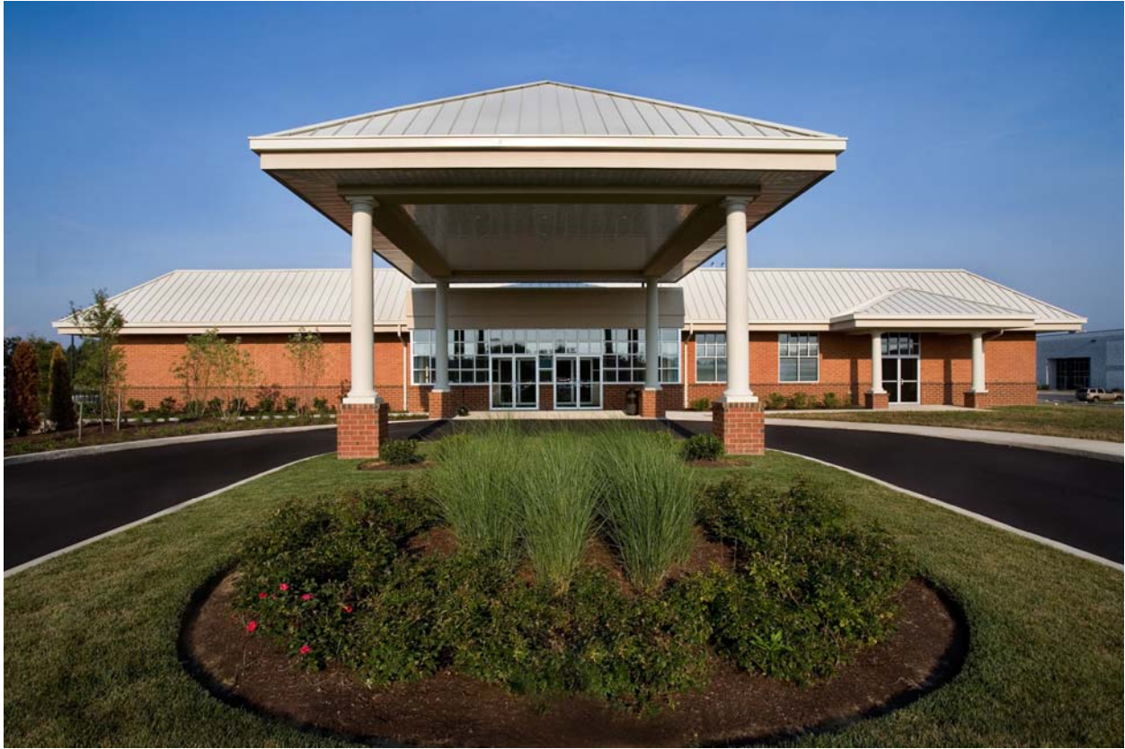
Plumbers and Pipefitters Local #74. Photo by Eric Crossan.
